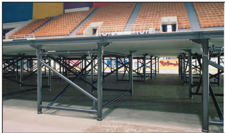
Large open spaces beneath the decks are ideal for stringing cables or stage-side storage.
